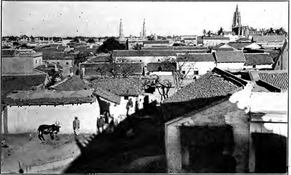
A GENERAL VIEW OF A CONGESTED INDIAN CITY WITH CLOSELY ABUTTING HOUSES
